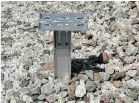
Fig. 5 – Mounting structure installed
